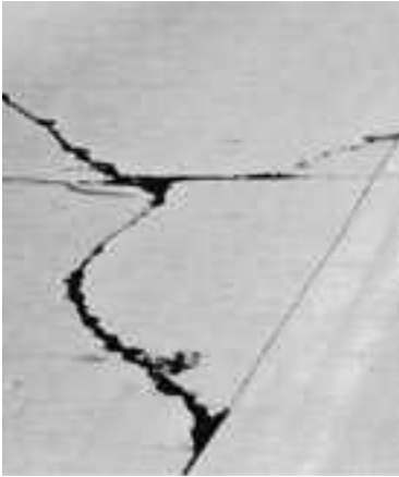
▼ Corner crack with spalling.
