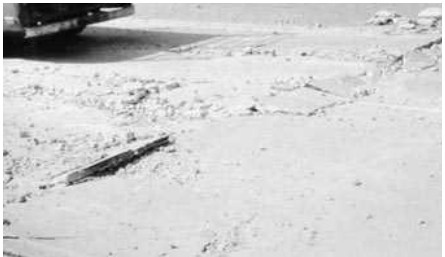
▼ A pavement blowup in progress. Concrete is crushed and slabs buckled.
