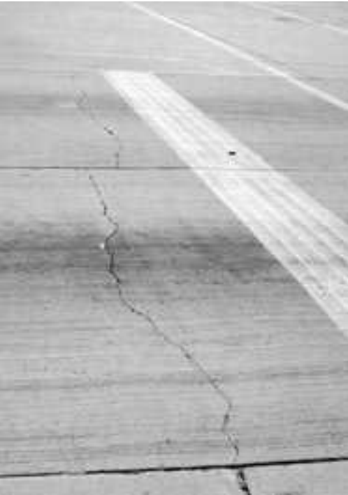
◀ Transverse crack. Tight, sound pavement.
