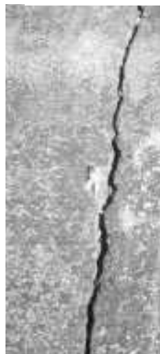
▼ Open crack, 1/2" wide; adjoining pavement sound.
