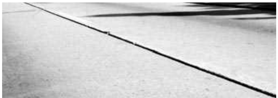
▲ Faulted longitudinal joint.
