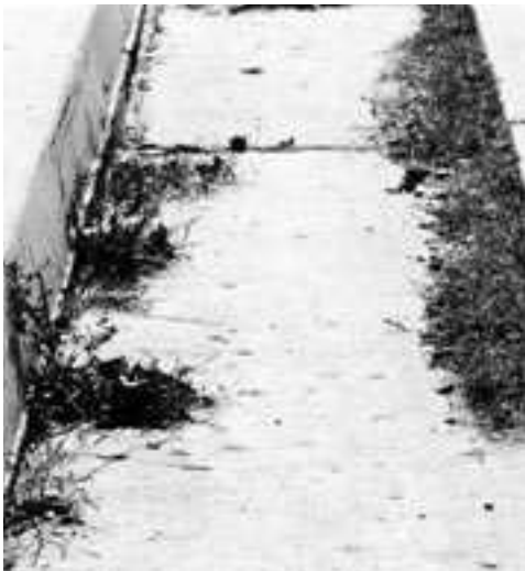
Extensive curb deterioration. Freeze-thaw damage to curb adjacent to inlet, and gutter is displaced. New curb and gutter are needed. ►
