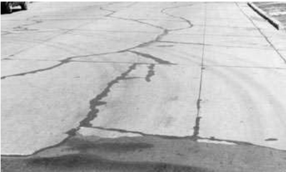
Extensive cracking and patching caused by settlement. Pavement was built on unstable sub-grade soils.
