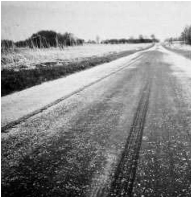
▼ Severe flushing.
