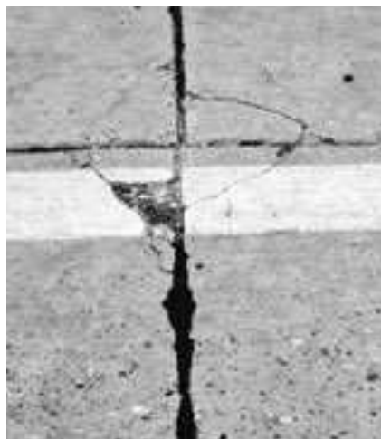
First signs of corner cracking.
