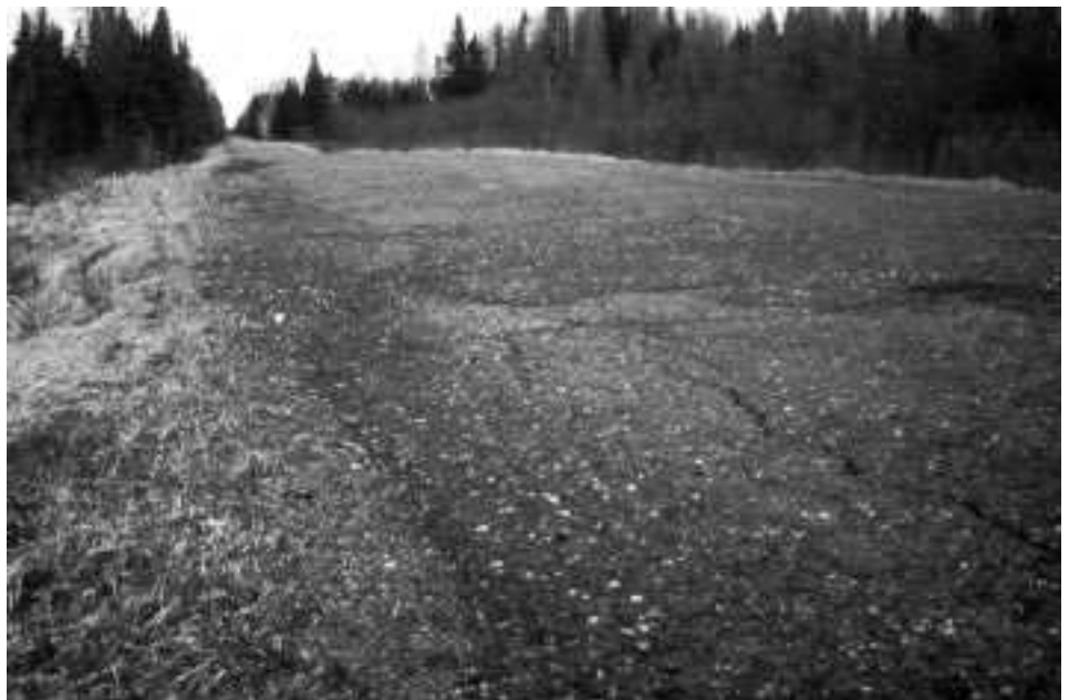
▲ Patches in poor condition, wheelpath rutting. Pulverize, strengthen and reconstruct.
