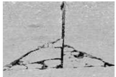
Corner cracking with broken concrete pieces.
