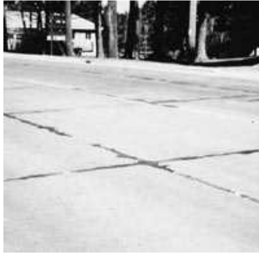
▼ Corner crack with spalling.
