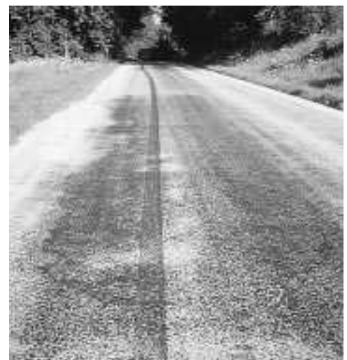
▼ Moderate flushing.
