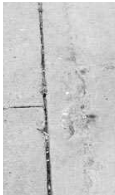
◀ Wire reinforcing mesh placed close to surface. Corrosion of the reinforcing steel causes the surface mortar to spall. Very difficult to patch and repair.
