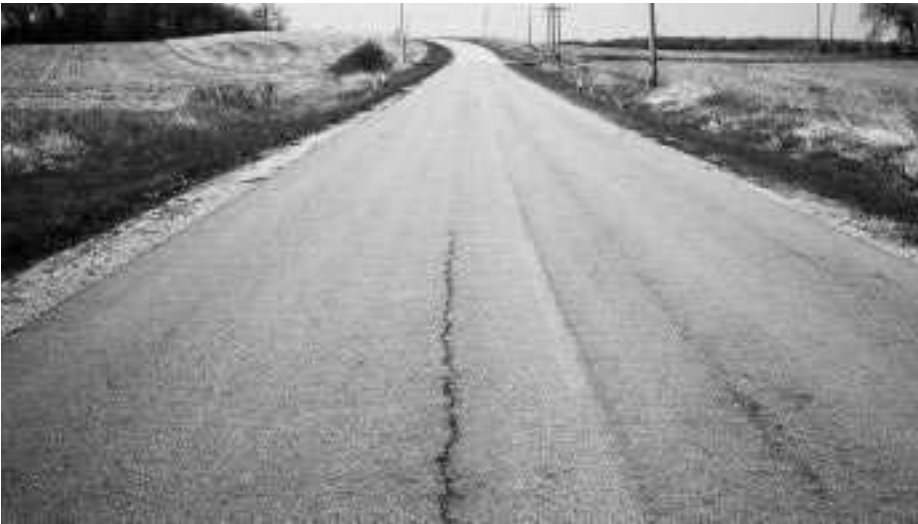
▼ Slight rutting; patch in good condition.
