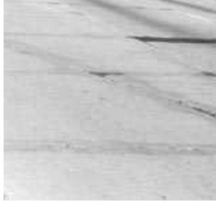
Surface discoloration near joints and cracks indicates D-cracking and severe slab deterioration.
