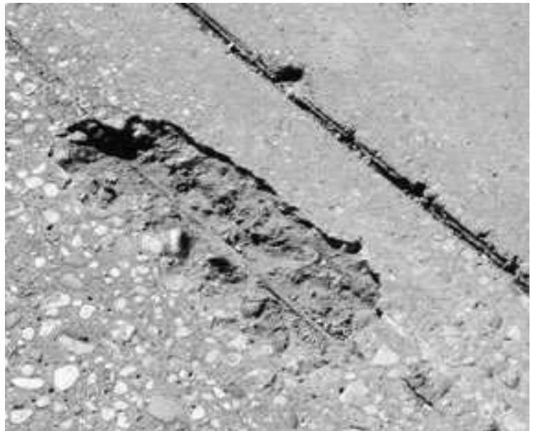
▶ Spalling over shallow reinforcing.
