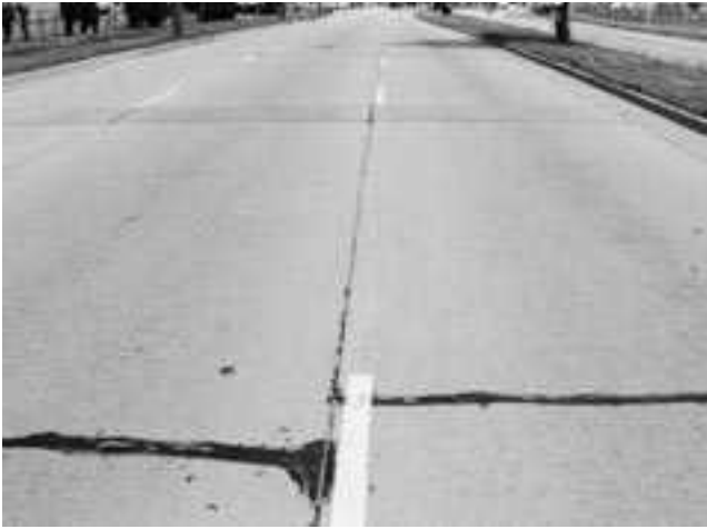
◀ Transverse crack. Tight, sound pavement.
