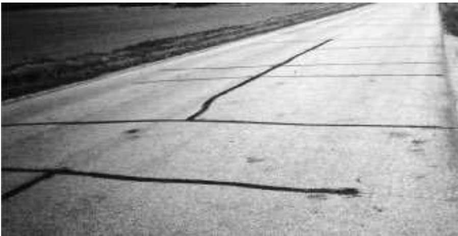
▼ Open crack, 1/2" wide; adjoining pavement sound.
