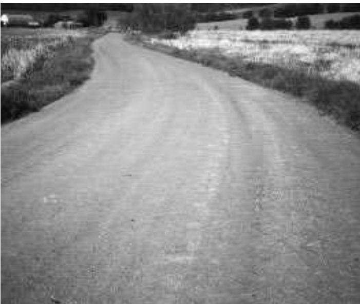
▲ New cold mix surface.
