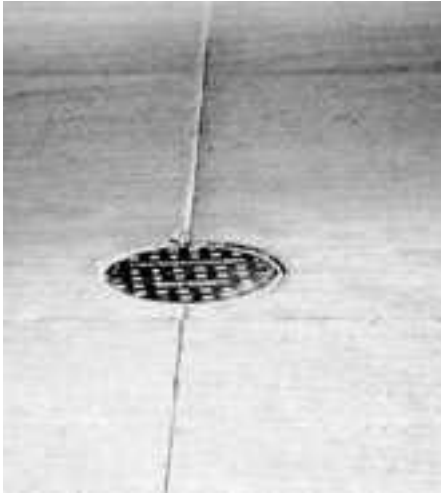
► Severe spalling of a transverse joint.
