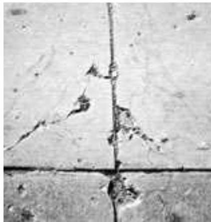
Corner cracking with broken concrete pieces.
