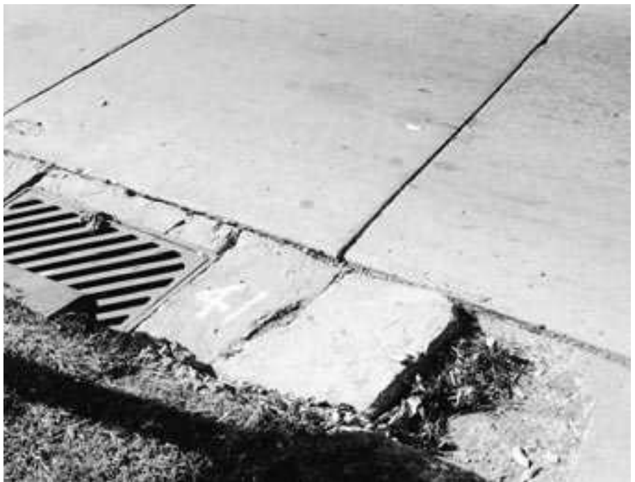
Extensive curb deterioration. Freeze-thaw damage to curb adjacent to inlet, and gutter is displaced. New curb and gutter are needed. ►
