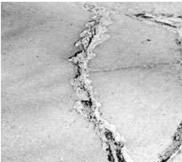
▶ Spalling over shallow reinforcing.
