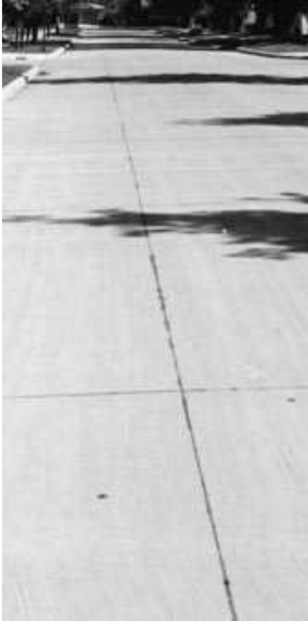
◀ New, well-sealed longitudinal joint.
