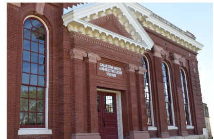
Renovated Galveston Water & Electric Light Building
